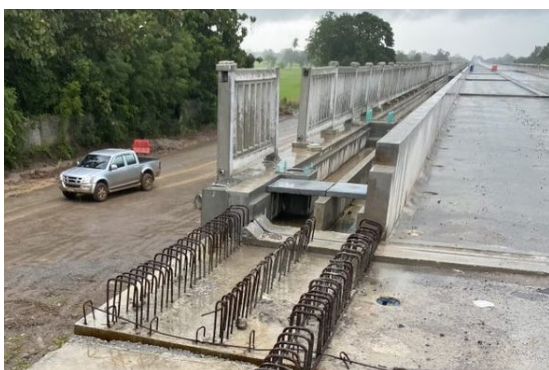
Picture-5 Duct at a boundary between viaduct section and embankment section
