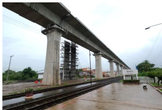
Picture-2 Viaduct 2 (near SRT Sung Noen station) with emergency stairs under construction
