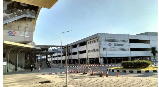
Picture 5: Pink line Min buri Station and Parking Garage building
