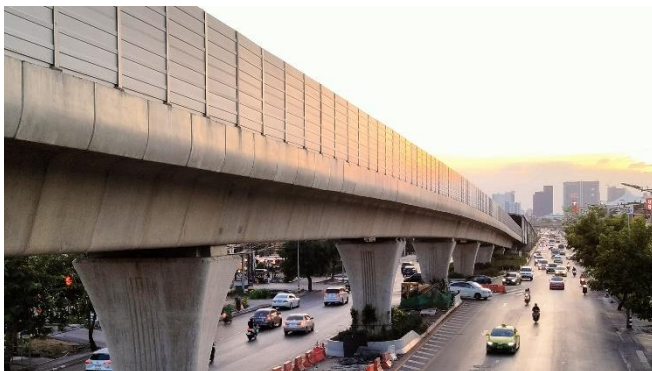
Picture 4 : Route transition to ground section before Sammakorn Station
